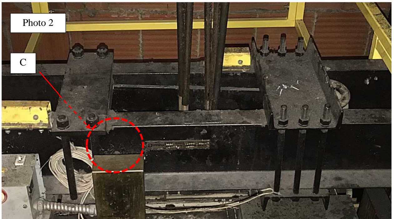
Photo 2 Overview of spring hitch arrangement
